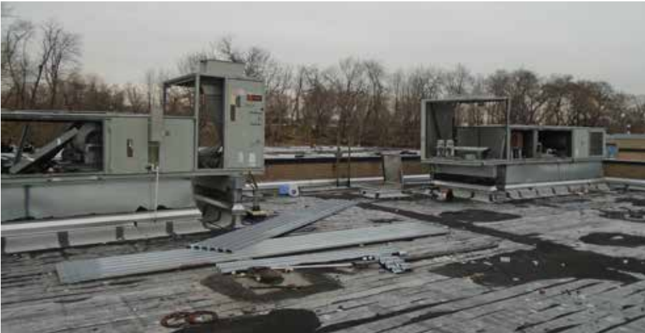
Views of Rooftop Mechanical Units
