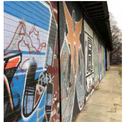
View of Exterior Wall
